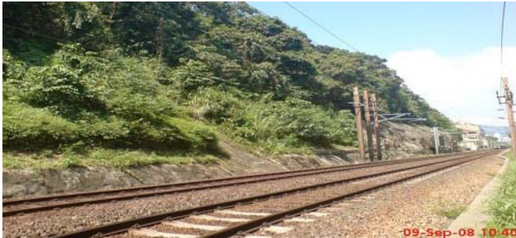
改善前 Before Improvement
