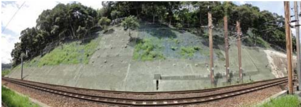
改善後 After Improvement
